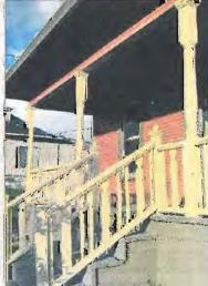
« Salvaged wood from other parts of the house was used to rebuild the porch and stairs. The porch columns were saved, and the railing got some decorative balusters.
